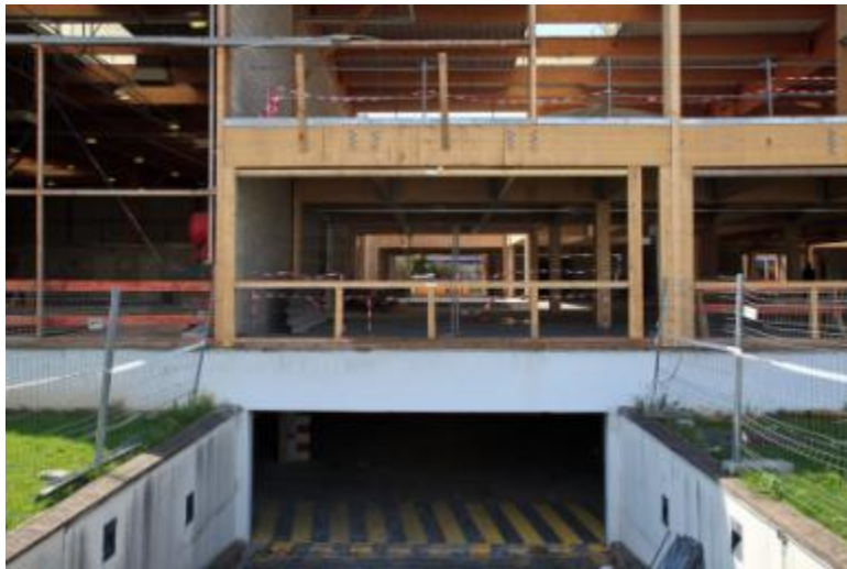
September 2011 – works in progress
