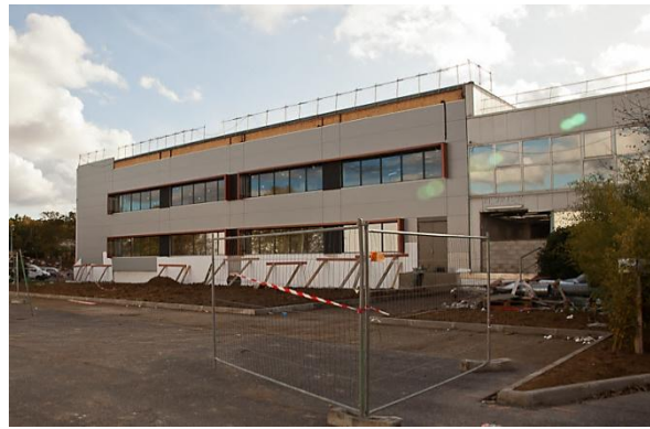
Installation of new Aquitaine facade
