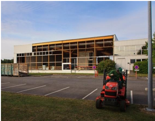
Aquitaine facade under demolition
